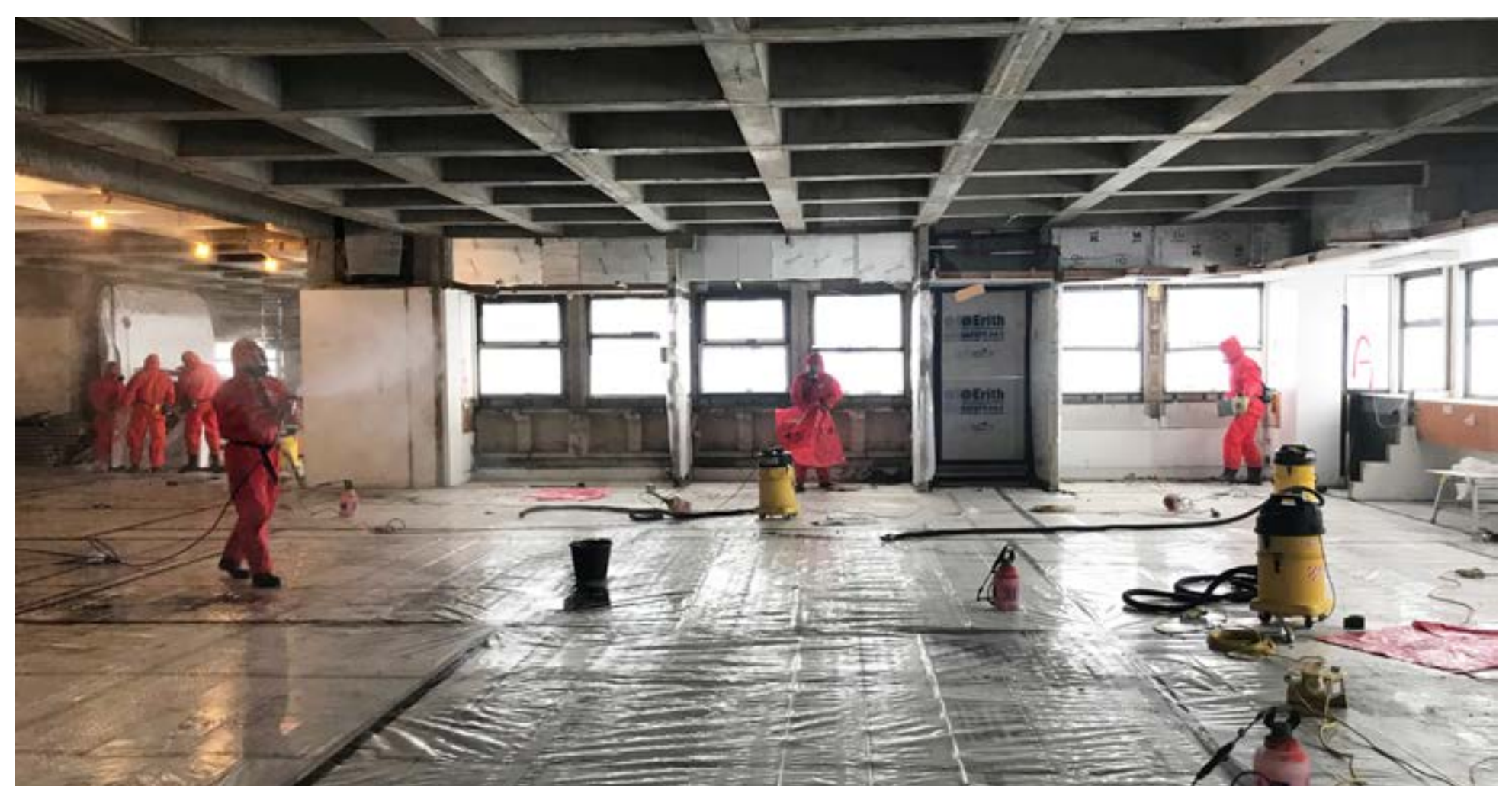
Erith removing ACMs under controlled conditions
