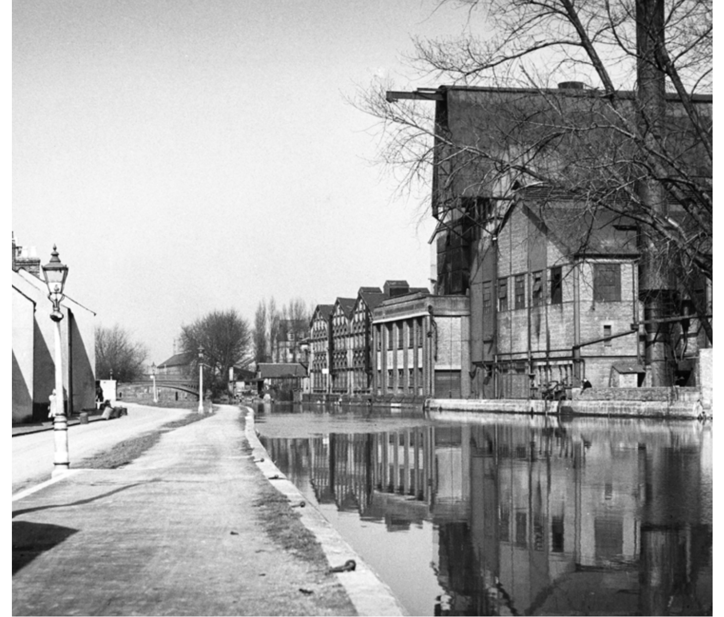
Osney Power Station in 1945
