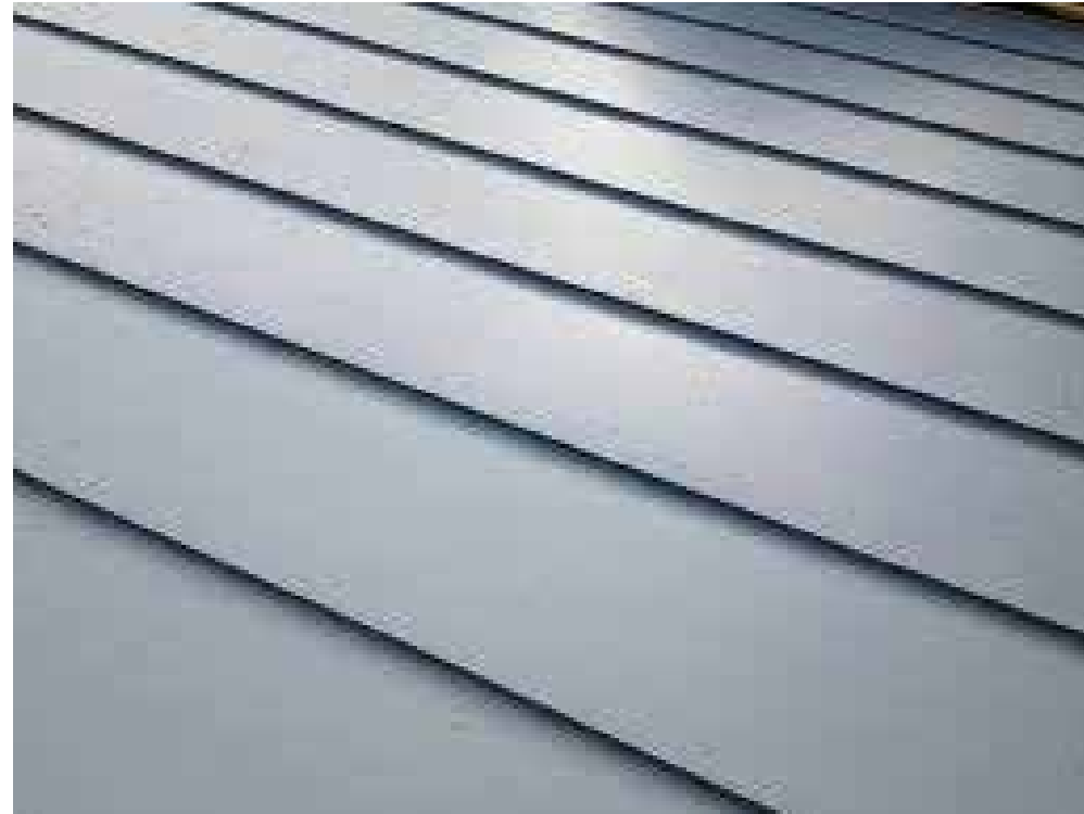
6 New standing seam roof finish
