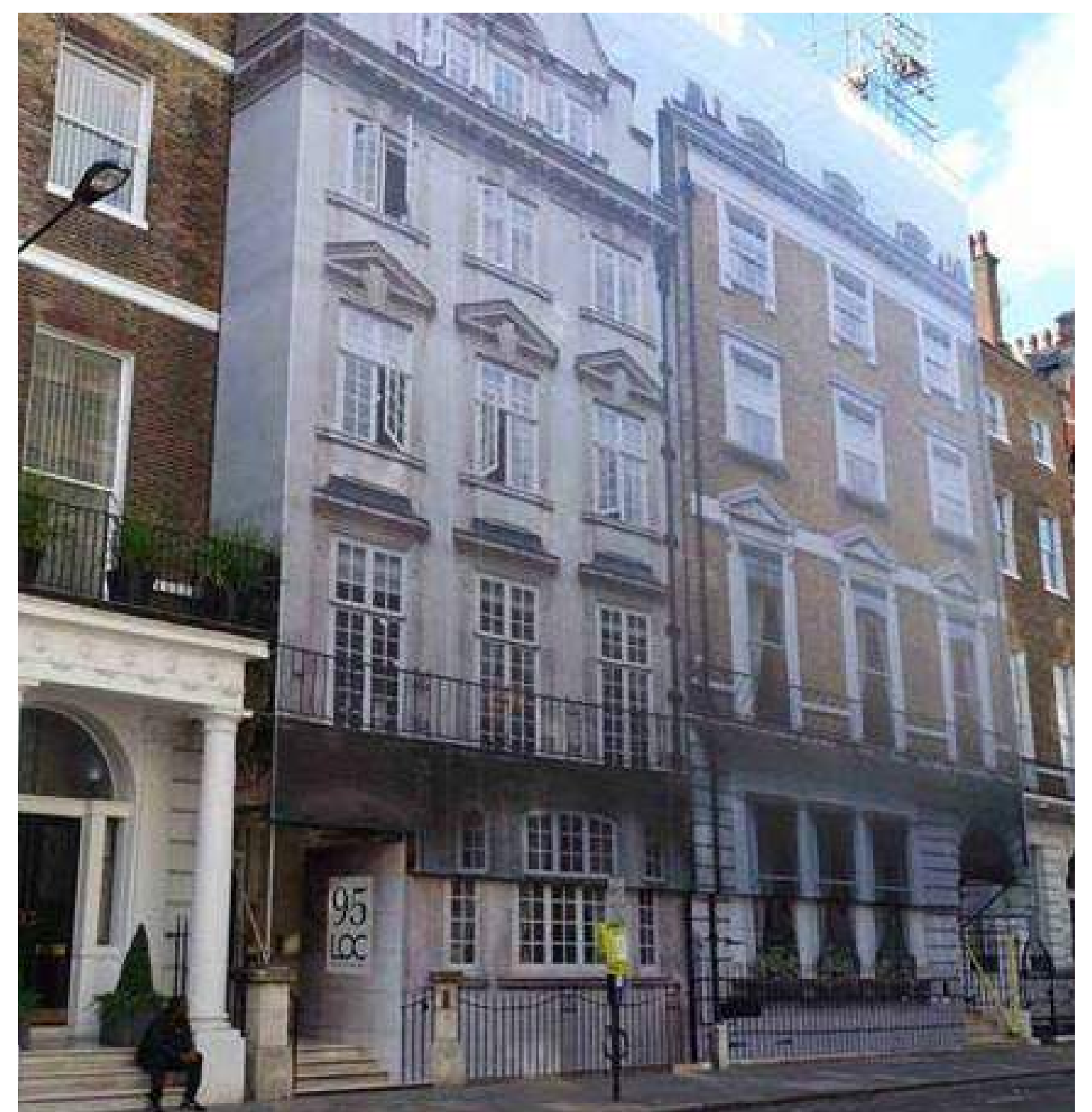
An example of a site where the scaffolding was wrapped to minimise the visual and acoustic impact of construction
